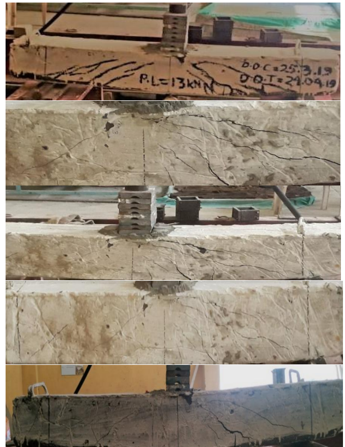
Fig.13. Crack pattern and failure mode for RCA as well as NCA based beams
