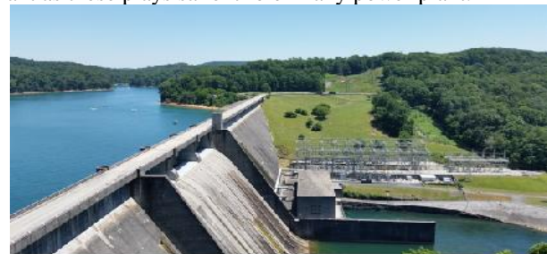
Fig. 13. Hydropower Plant site
