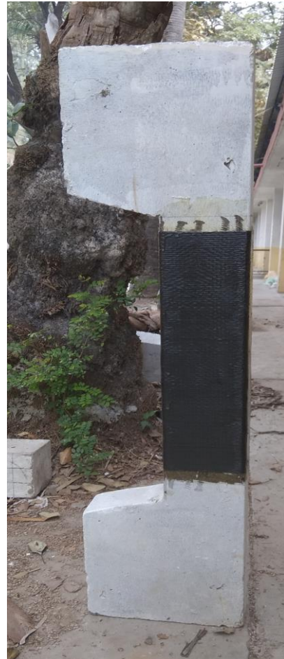
Fig 4. Reinforced concrete columns Wrapped with CFRP source: currently used
