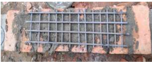
c) Mesh type reinforcement
