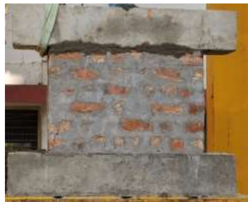
Figure 10: Unreinforced Brick Wall
