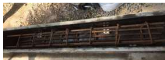
a) Mould with steel reinforcement
