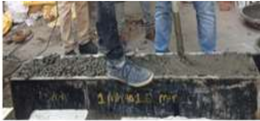
b) Casting of Beams
