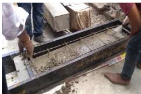
Fig. 8: The casting of conventional reinforced concrete beam
