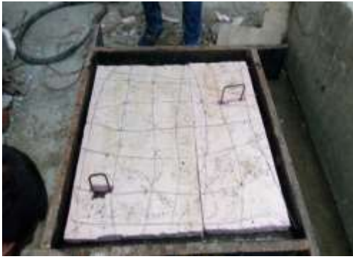
Fig. 4: Sandwich slab
