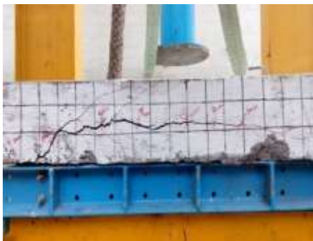
Fig. 11: Cracks on the slab after loading
