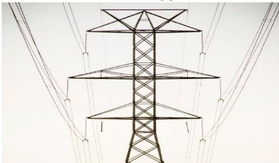
Figure 3: A Transmission Tower
