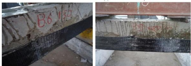
Figure 3.4 Carbon fiber Retrofitted beam with resins (ISO, Epoxy, GP)
